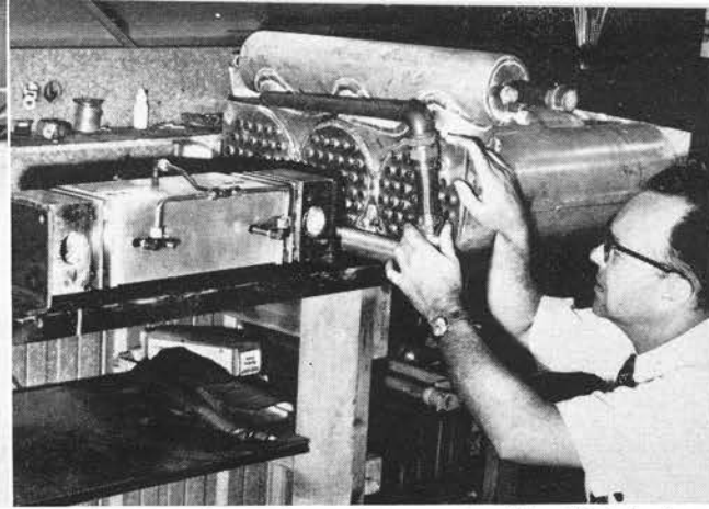
Heat recovery and vaporizer unit is examined by Chief Engineer Leonard Keller. Refrigerant flashes into gas and is reheated by burner exhaust here. Box on left is the boiler feed pump.
