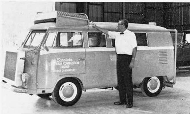
Inventor Wallace L. Minto points out rooftop condenser for ancient Stanley Steamer engine, driven by refrigerant fluid, that powers this VW minibus. Vehicle was a test bed to prove theory.
